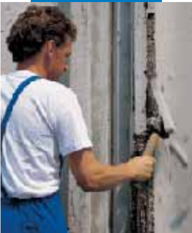
Demolition of degraded concrete
