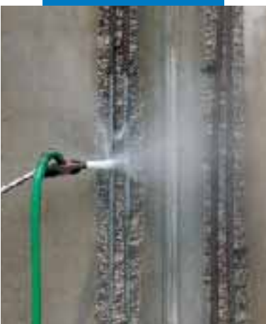
Cleaning reinforcing rods
