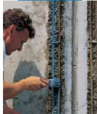
Application of Mapefer
