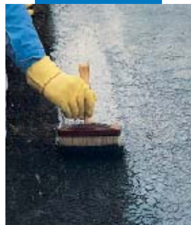
Applying Primer for Aquaflex over an existing asphalt membrane
