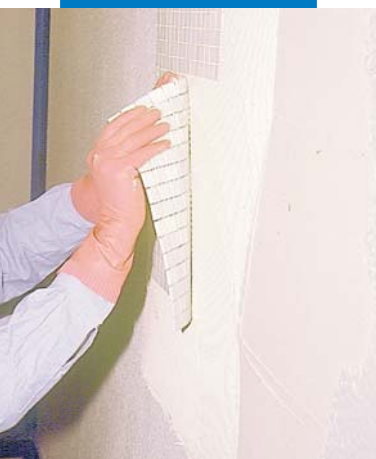
Laying glass mosaic
