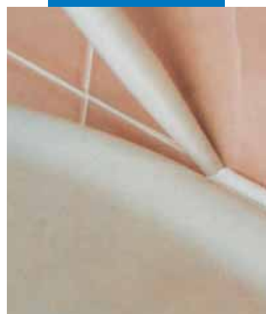
Sealing sanitary ware
