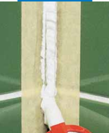
Application of Mapesil AC
