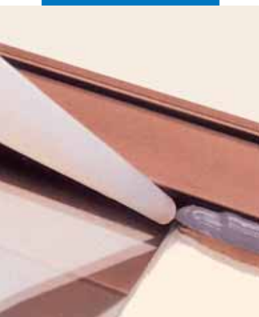
Sealing aluminium window frame with Mapesil AC
