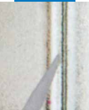
Sealing U-profile glass
