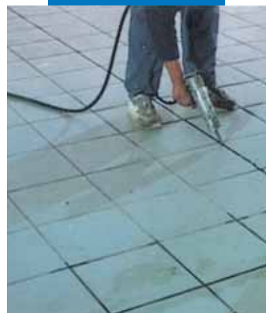
Sealing ceramic tile floor with Mapesil AC
